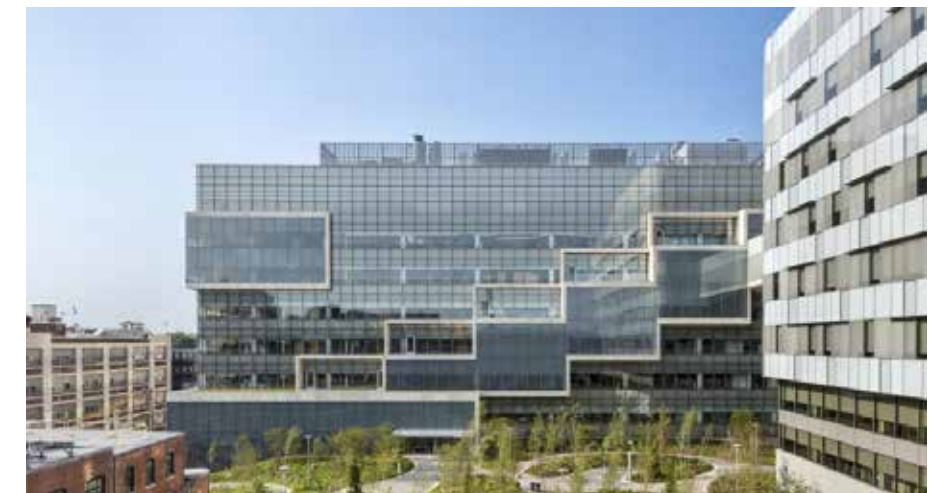
SINGLE-TENANT BUILDINGS Novartis building at Kendall Square Cambridge, Massachusetts, United States
