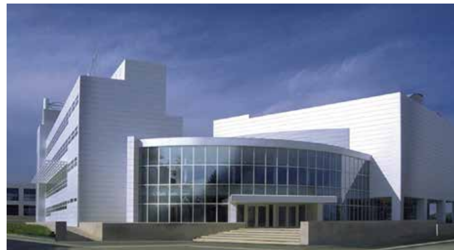
ICONIC CENTRAL BUILDING San Sebastian Science Park San Sebastián, Spain
