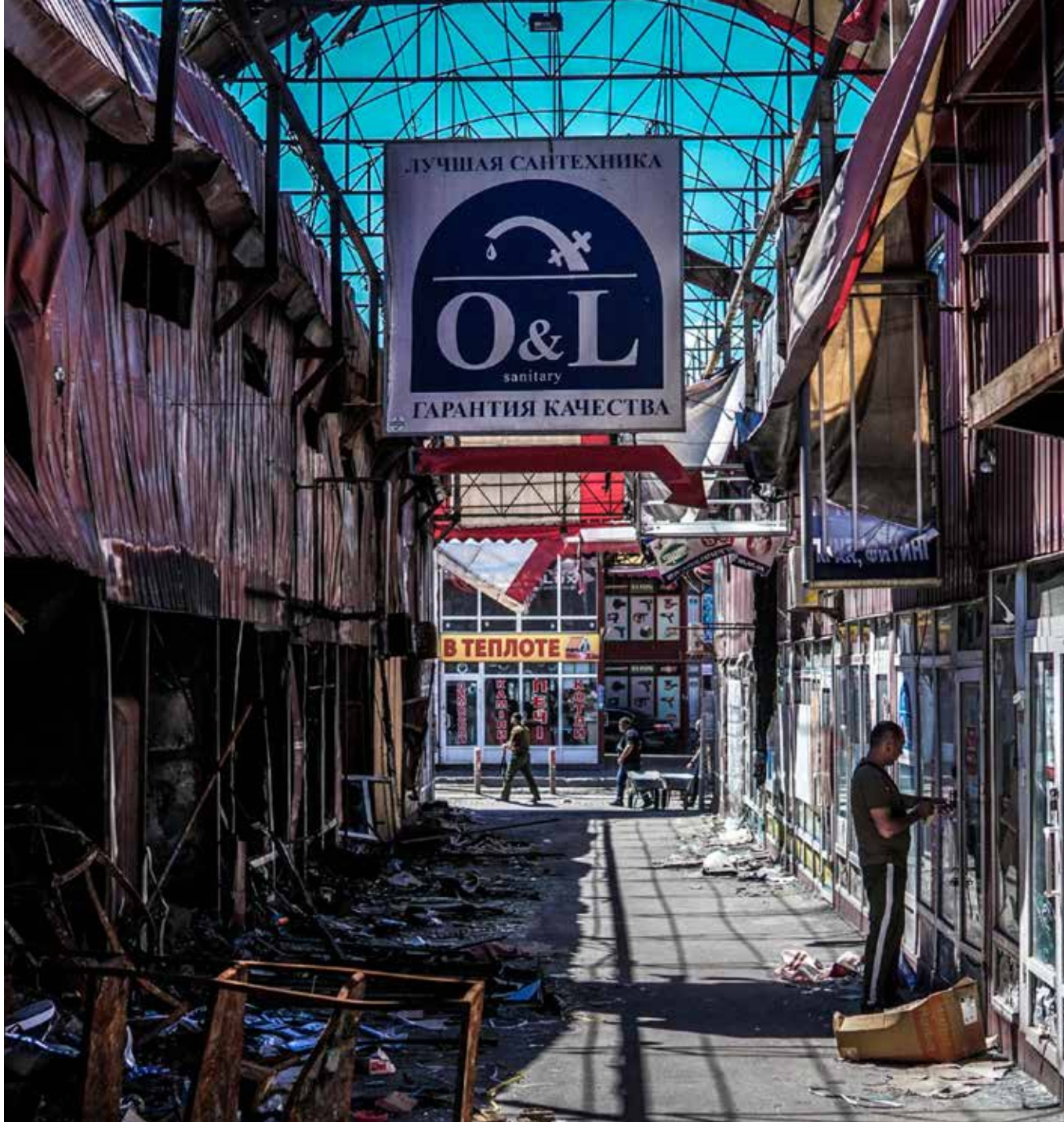
Interior image of the damages at Barabashova Market
